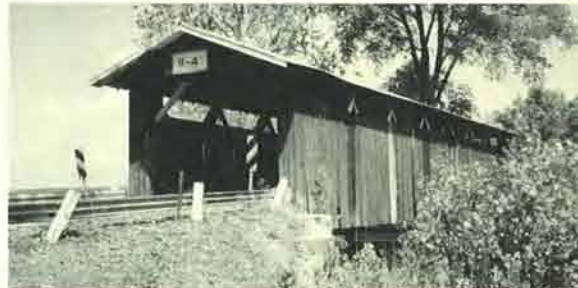
Ballard Road Bridge
