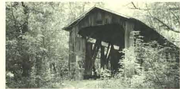
Glen Helen Bridge
