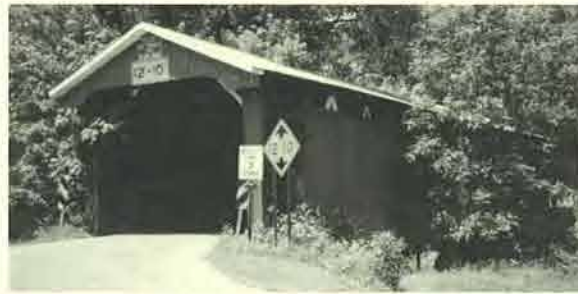
Stephenson Road Bridge
