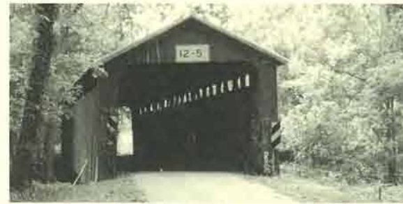
Charleton Mill Road Bridge
